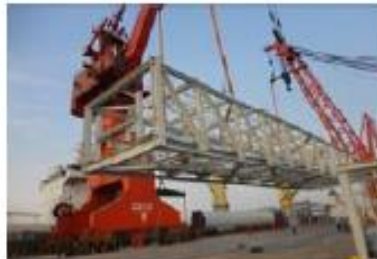
Steel Construction 钢结构
